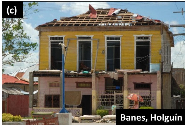
Figure 28. a) House in Holguín destroyed by Sandy's strong winds, b) severe structural damage in Holguín, c) roof damage to a residence in Holguín, and d) storm surge flooding at the Hotel Baconao near Santiago de Cuba. Images courtesy of the Cuban Meteorological Service.
