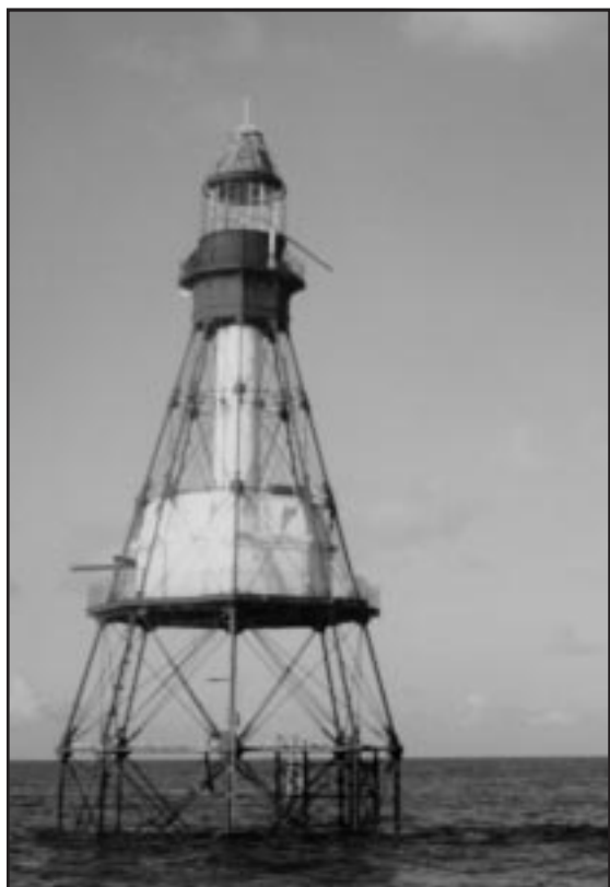
Fowey Rocks C-MAN station before Hurricane Andrew.
