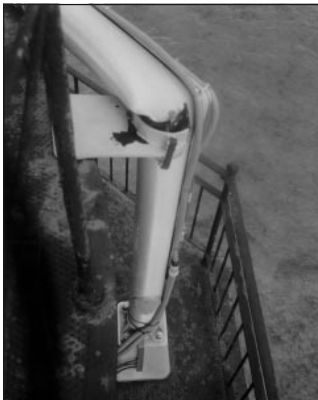
Fowey Rocks trolley mast bent 90° by Hurricane Andrew.
