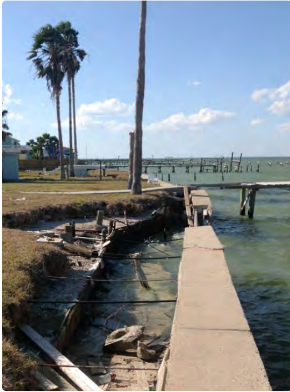
Bulkhead failure leads to erosion and land loss. Photo: Texas General Land Office
