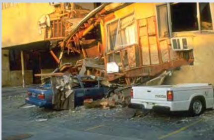
The first story of this apartment building collapsed, crushing cars below (FEMA photo).
