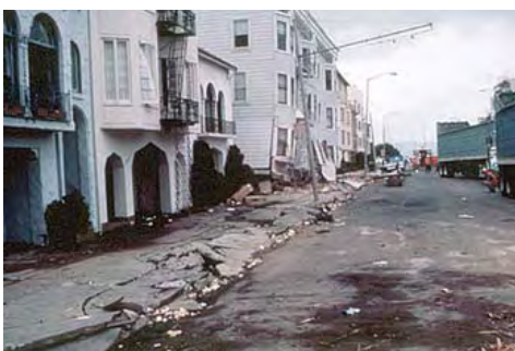
Sandy soils can shake so much that they liquefy, causing buildings to sink and buried pipes to break. In steep hilly terrain, landslides can also be triggered (USGS photo).
