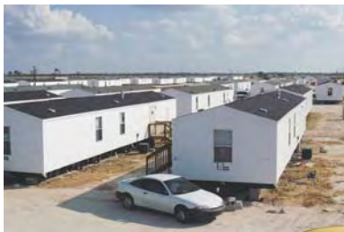
FEMA mobile homes were used to provide temporary housing after Hurricane Charley in 2004. Nearly a year later, these trailers were still being used. (FEMA photo)
