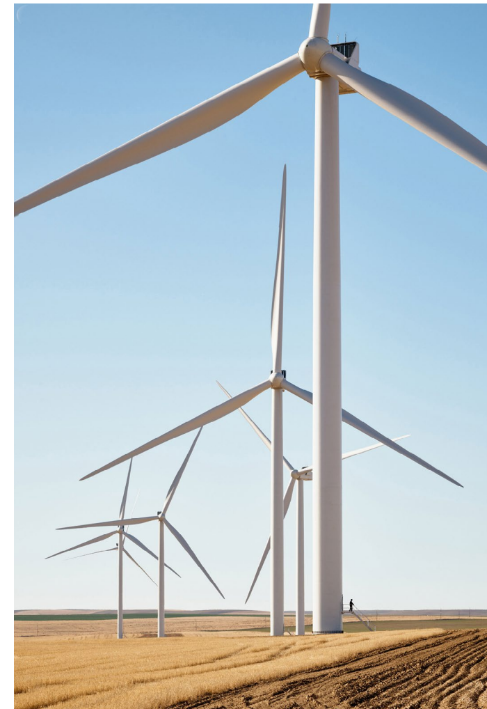
At 200-megawatts, the Montague Wind Power Facility in Oregon is one of Apple's largest renewable projects to date.
