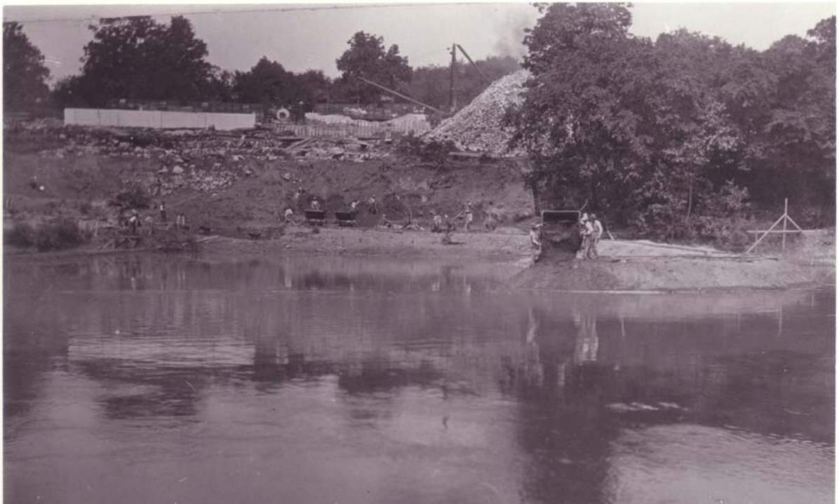
6/14/1910 – View from east bank showing method of building coffer dam from earth excavation from wheel pits.
