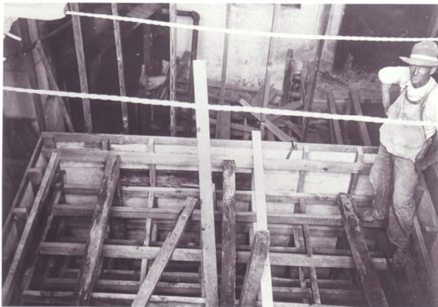
9/6/1911 – 1750 KW turbine foundation.
