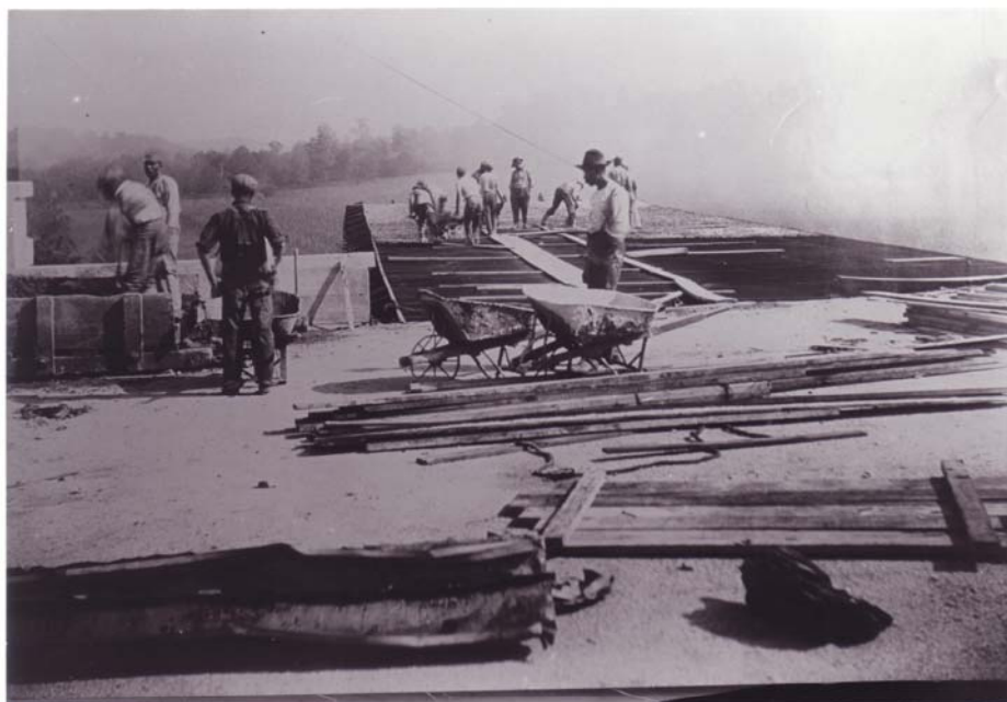
9/29/1911 – Concreting roof slab. Water wheel building.
