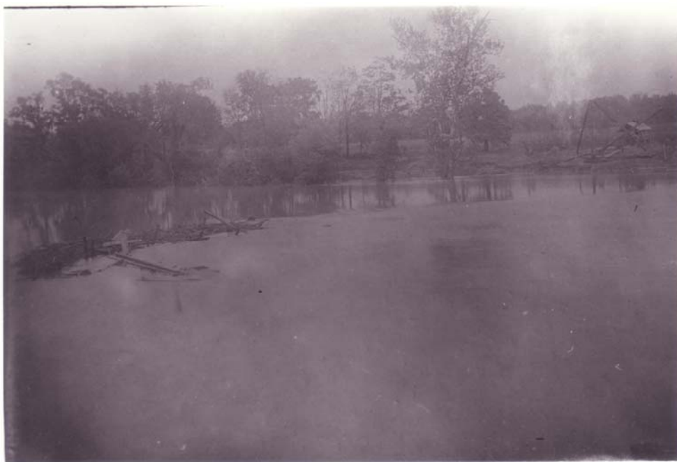
1910 – Williams Historic dam, construction photograph.
