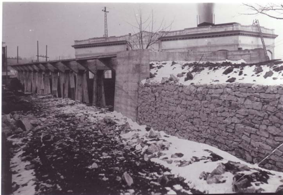
2/14/1912 – View of coal trestle from south end also showing abutment and dry well.
