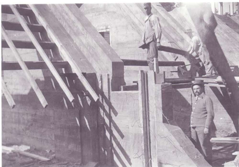
1910 – Williams Historic dam, construction photograph.
