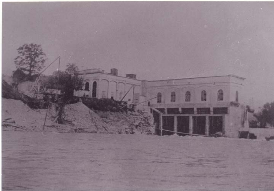
1910 – Williams Historic dam, construction photograph.
