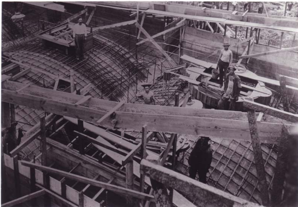
8/17/1911 – Reinforcement thrust bearing floor from pouring tower.
