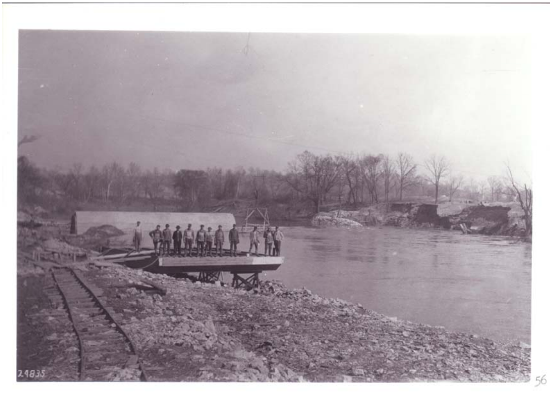
2/15/1911 – View of dam and pile driver boat.
