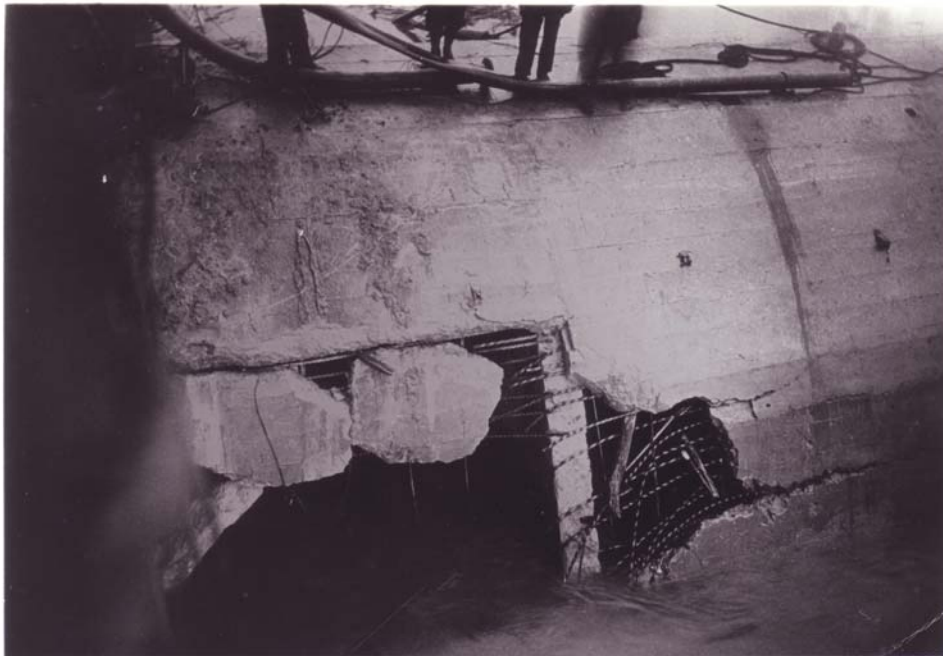
12/31/1911 – Showing damage by log to downstream side of first bay of dam.
