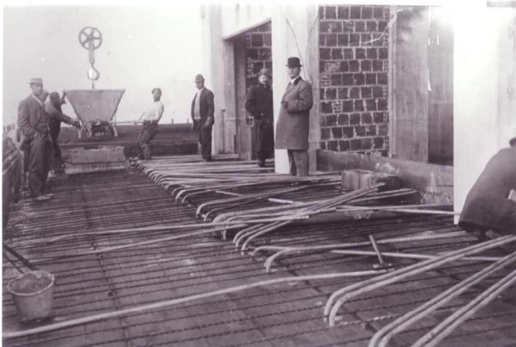
11/20/1910 – Roof of remote control room. Conduits and reinforcement in place.
