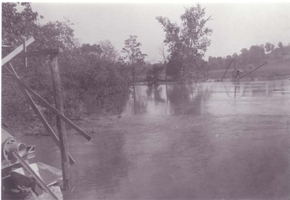
1910 – Williams Historic dam, construction photograph.
