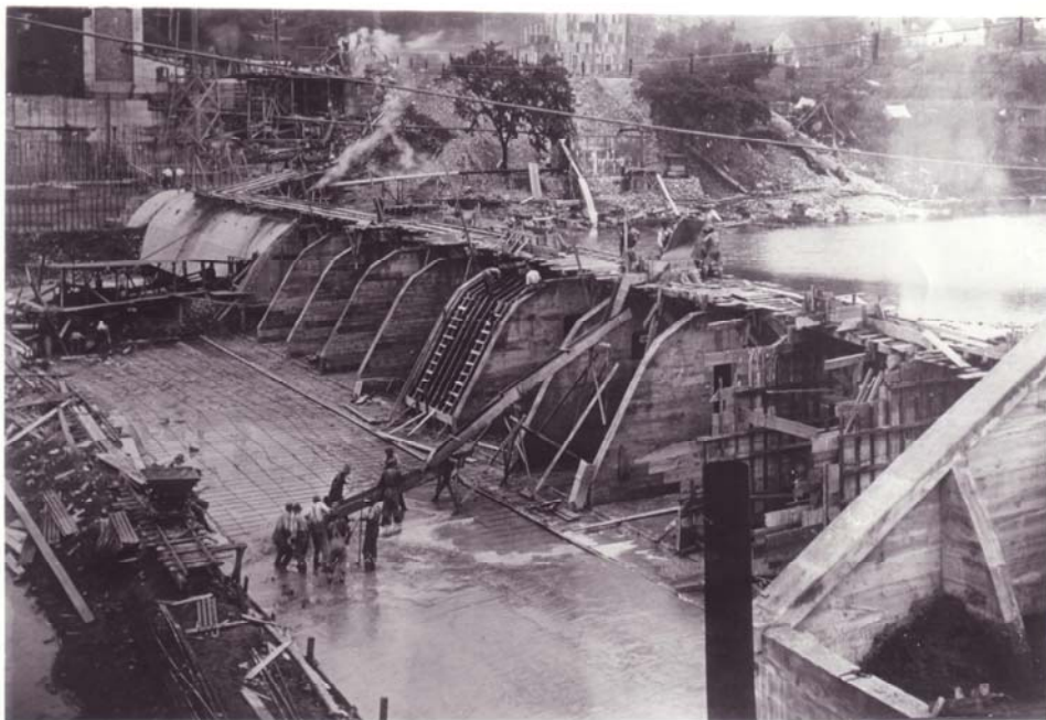
8/2/1911 – Concreting top of mattress, apron coating.
