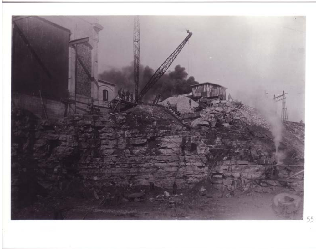
2/15/1911 – View of wheel pit excavations.
