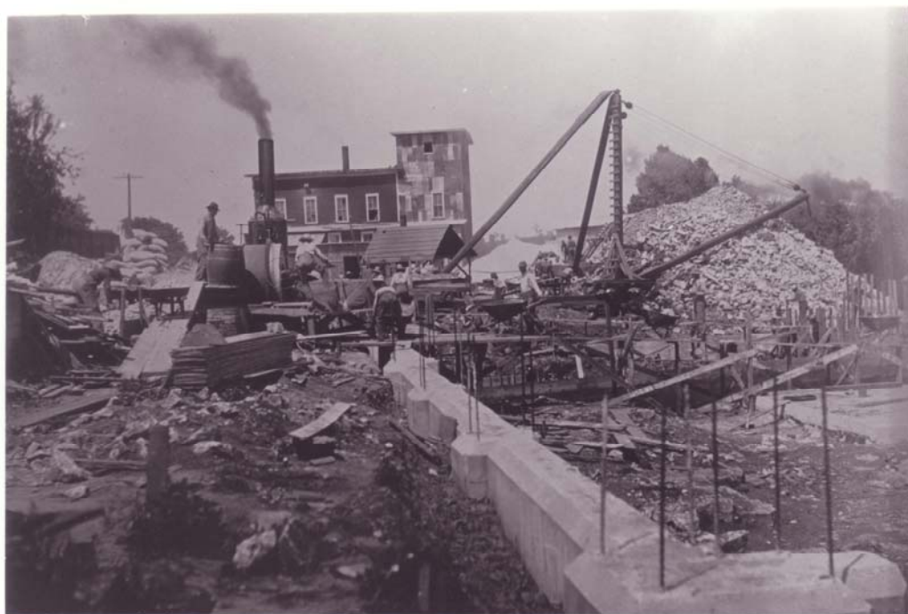
6/21/1910 – Concreting walls in basement of engine room. View from southwest corner of boiler room.
