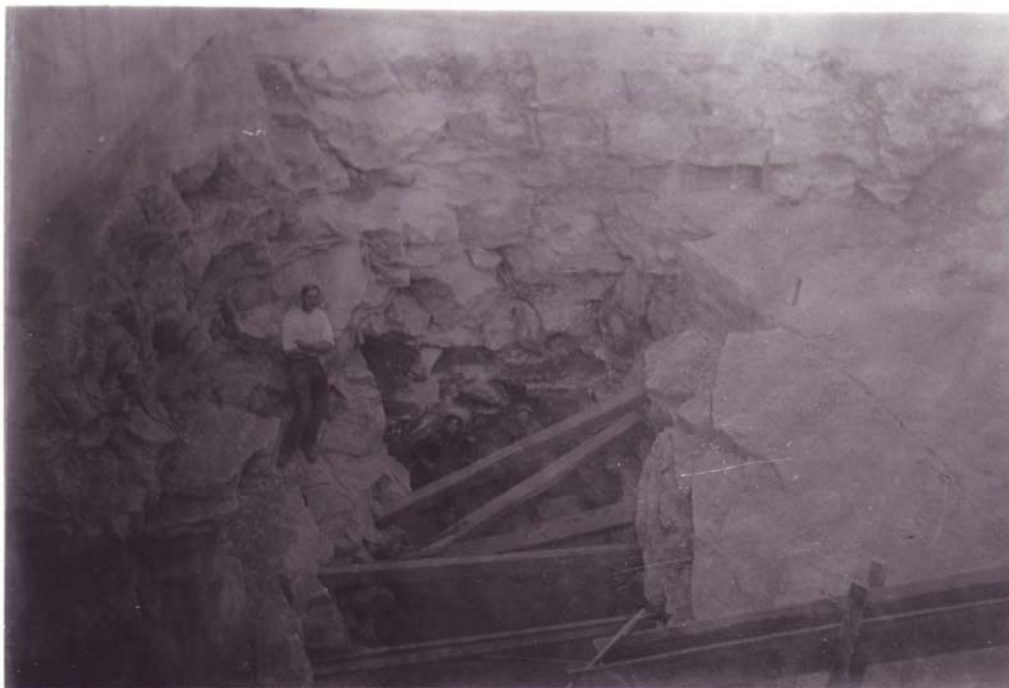
1910 – Williams Historic dam, construction photograph.
