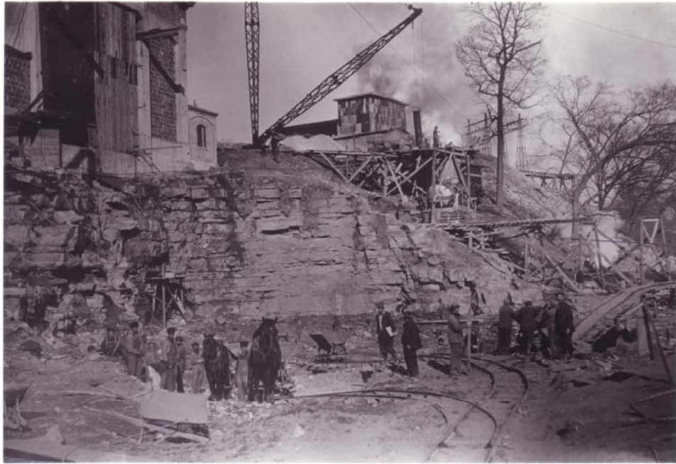
11/29/1910 – Wheel pit excavation and tram track around dam.
