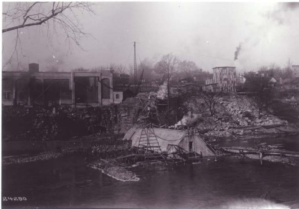
12/21/1910 – View of work from opposite side. Tram car on trestle over coffer dam to east bank. Forms in place for tunnel openings.
