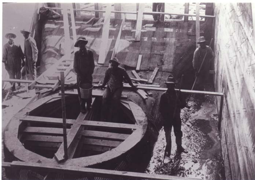
8/31/1911 – Concreting lower draft tube #3.
