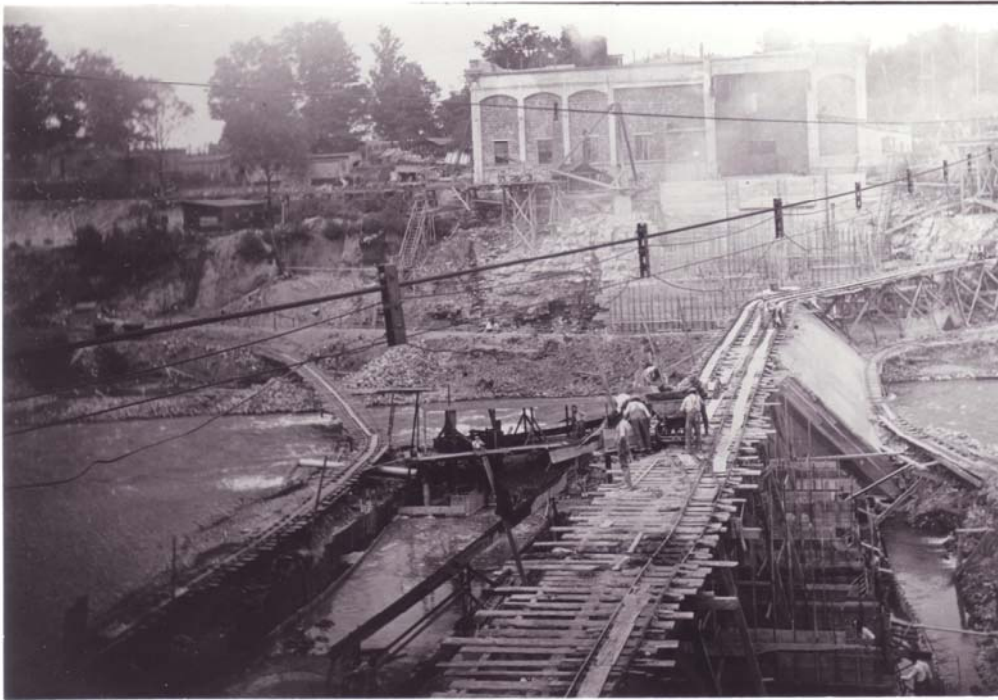
7/25/1911 – Concreting mattress of dam, showing buttress forms.
