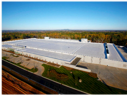
Maiden data center
