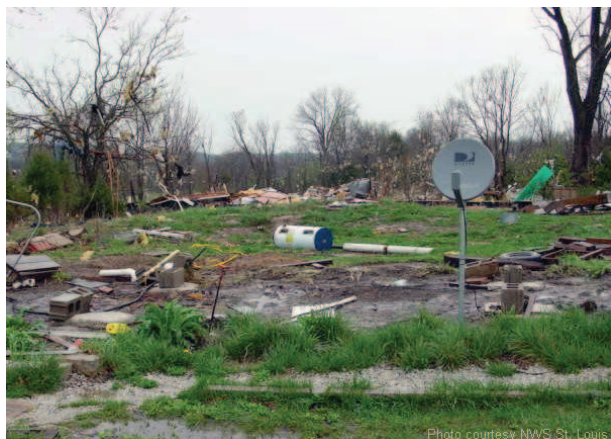
FIG. 2. Site of the fatal destruction of a mobile home near Fulton, Missouri, by a rain-wrapped, F1-rated tornado on 10 Apr 2001 (for meteorological documentation, see Glass and Britt 2002). At DoD 9 (complete destruction of unit), anywhere from EF1 to EF3 can be assigned for this DI in EFkit. The lack of damage to surrounding trees and to the adjacent satellite TV receiver may indicate either weaker winds than apparent (rating potentially as low as EF0) or the presence of a small-scale subvortex with winds at or above the EFkit default level of EF2. Uncertainty therefore yields a four-category margin of error in this scene alone. (Photo courtesy of NWS St. Louis.)
